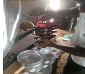
Figure 56. Riveting of the various components arrangement of components on the frame for marking before riveting
