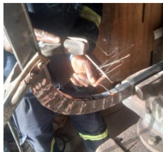
Figure 46. Welding the curved part of the frame
