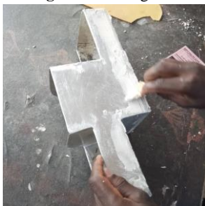
Figure 52. Application of the filler
