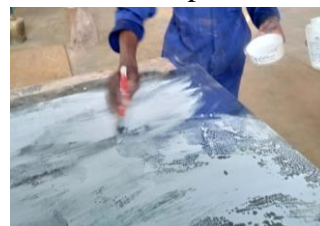
Figure 25. Application of the glue on the metal surface
